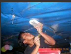
Installation of Solar LED Light
