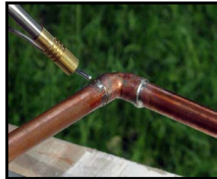
Figure 21. Heating and applying solder
