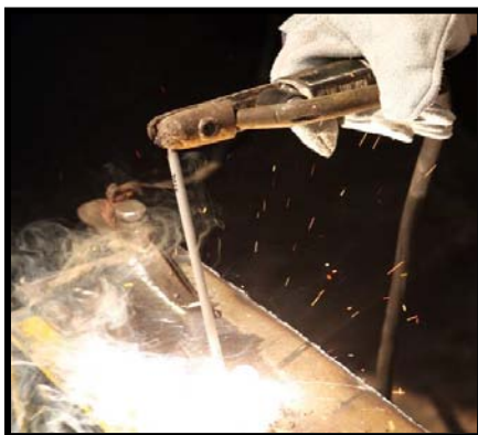
Figure 22. Metal stick welding
