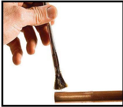
Figure 20. Applying flux to joint
