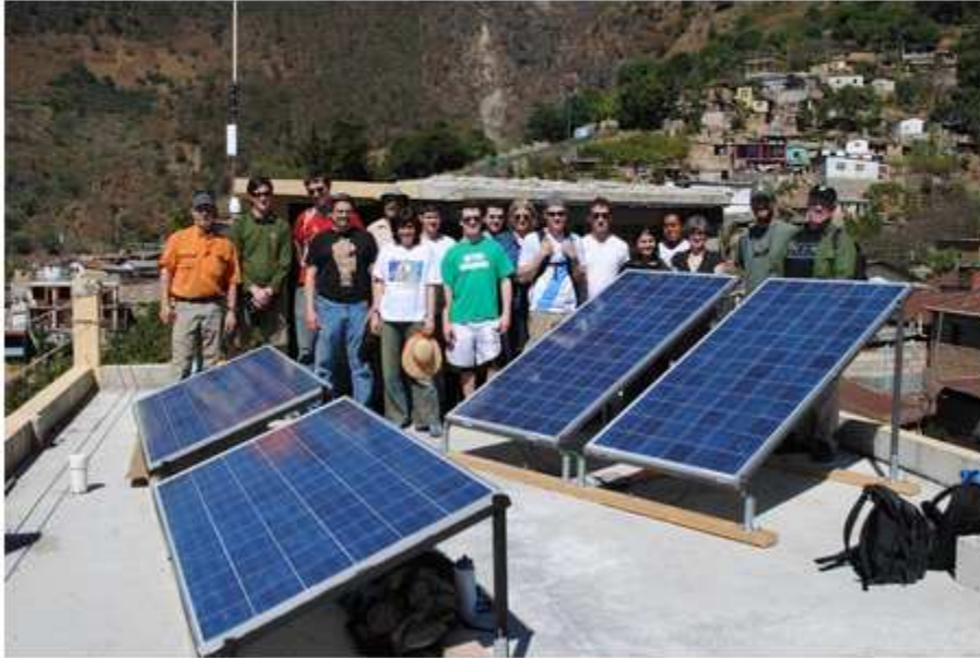
Santa Cruz Solar – Installation Team
